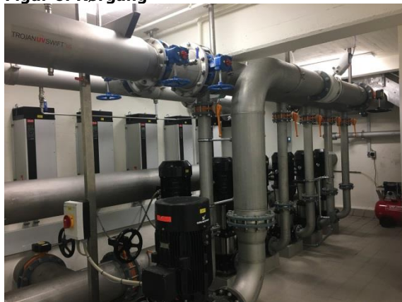
Figur 8: Rentvandspumper
